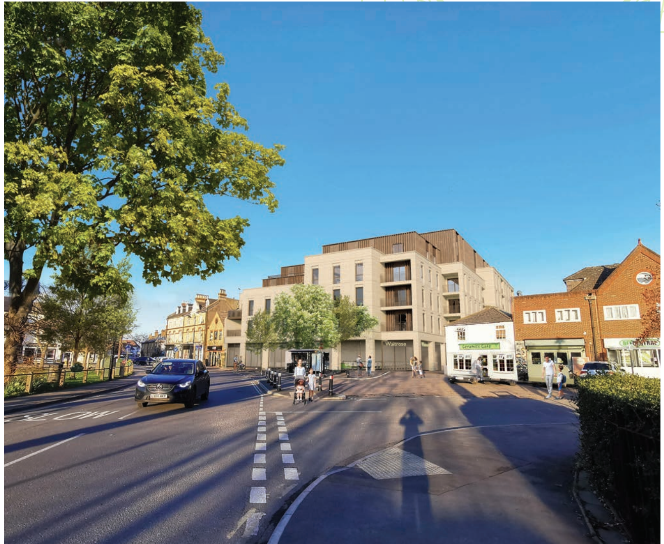
Image showing the new scheme from Burwood Road
